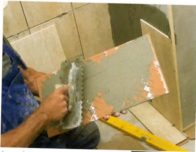
Successful installation of large format tiles includes: using the appropriate sized notched trowel; burning of the adhesive into the substrate; and backbuttering of the tile with the adhesive.
