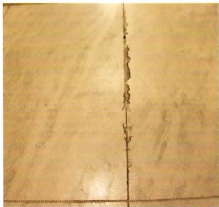
Tile produced on a faster production line will twist and warp.
